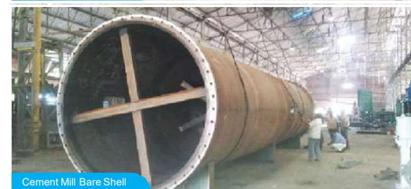
Cement Mill Bare Shell
